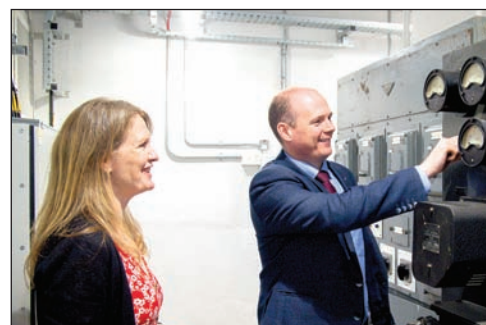
Communities Minister Gordon Lyons and Rhonda Robinson, Department for Communities archaeologist examines the restored generator at the Belfast War Rooms. The War Rooms is the new archive facility for the Historic Environment Record of Northern Ireland (HERoNI).
