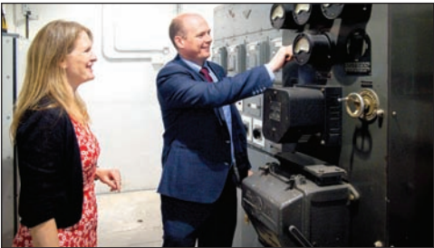
Communities Minister Gordon Lyons and Rhonda Robinson, Department for Communities archaeologist examines the restored generator at the Belfast War Rooms. The War Rooms is the new archive facility for the Historic Environment Record of Northern Ireland (HERoNI).
